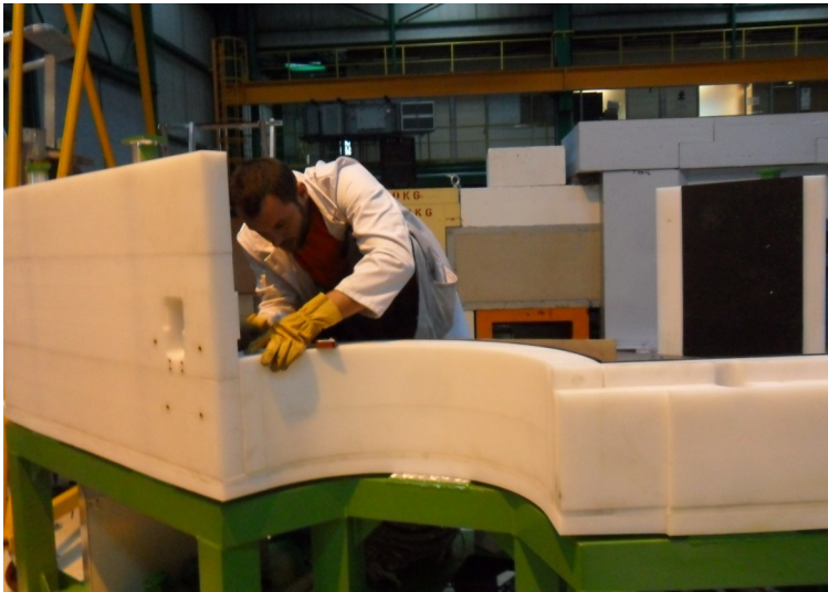
Figure 2: Pre-assembling the polyethylene protection in the guide hall
